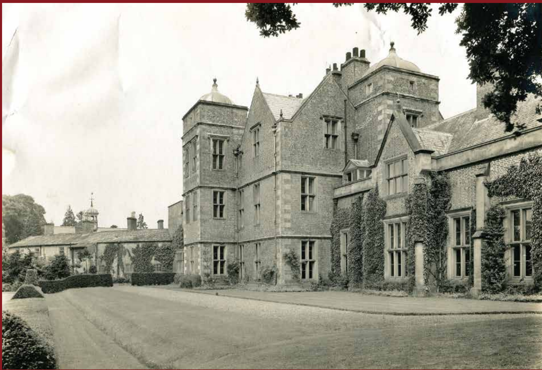
This photograph from the 1890s or 1900s shows the Hall from the southwest. The Carpenters added the gothic-style drawing room (later the library) on the right in 1818.
