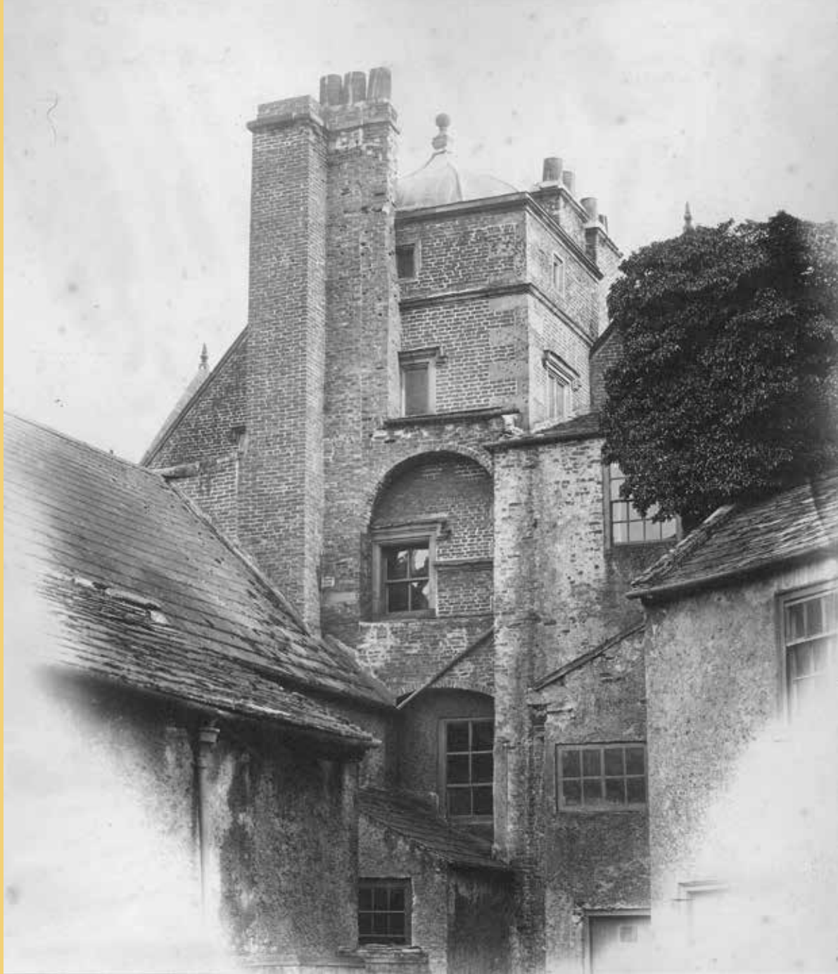
The Service Wing was built by the Crowes in the 1700s. This photograph from 1867 shows how the Service Wing was attached to the north tower of the Hall.
