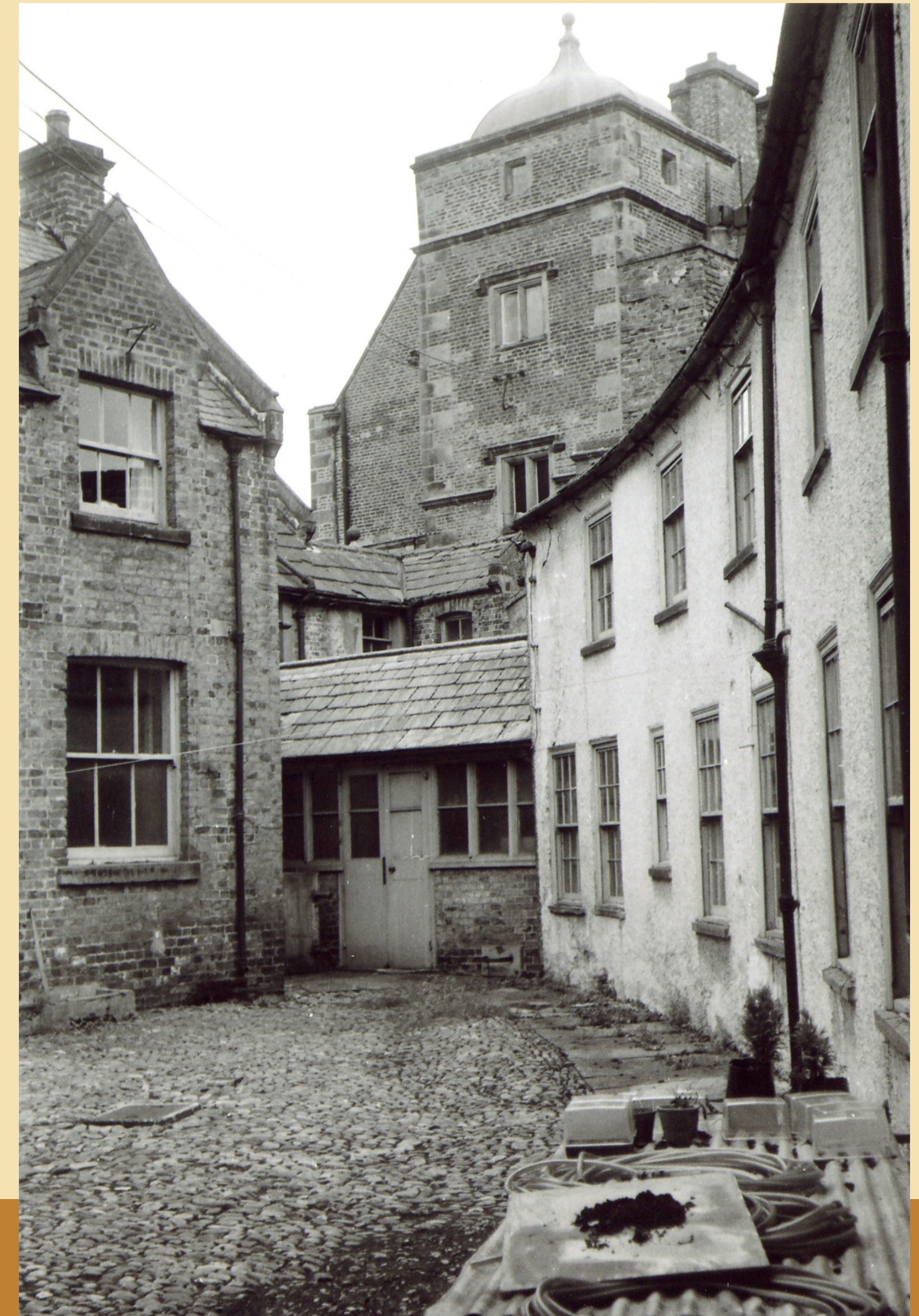
In the 1970s most of the unsound service wing was demolished so that the rest of the Hall could be saved.
